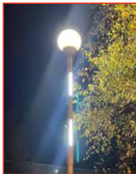
Illuminated refuge post extension
